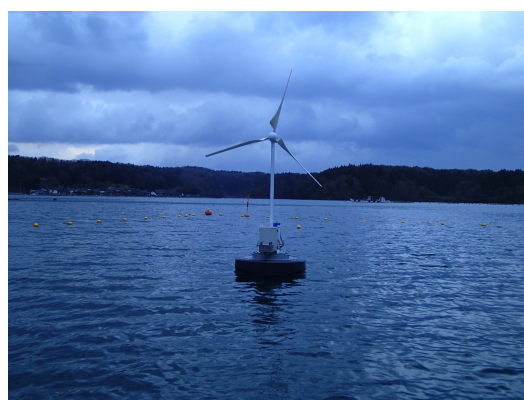
(f) Wind turbine after the installation work
