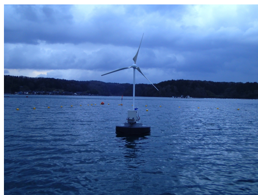
(f) Wind turbine after the installation work
