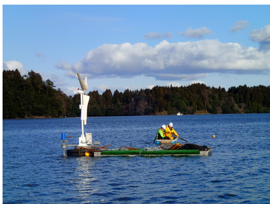
(e) Connection of the mooring chain
