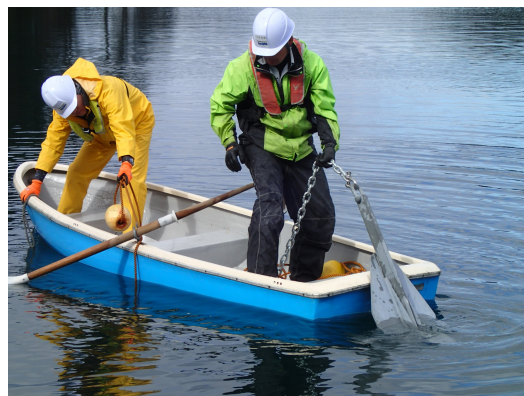
(b) Installation of the anchor
